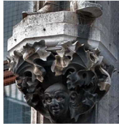
Figure 3: Photo of a polluted object: white zones are washed by rainfalls or strong flows and remain protected from darkening, while the black zone is covered by pollution particles trapped into gypsum.
