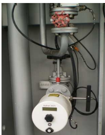
Obr. P2 - 6: Hydran sensor
