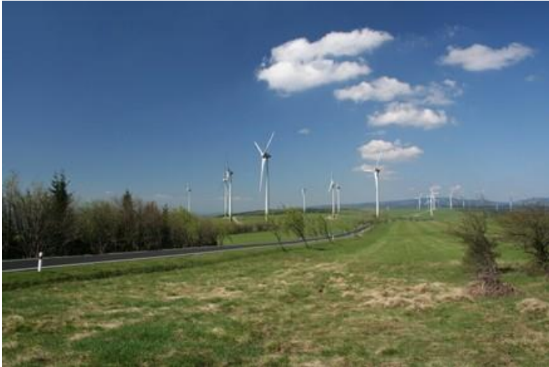
Obr. 1 Farma VE Kryštofovy Hamry, 21 turbín, 42MW [18]
