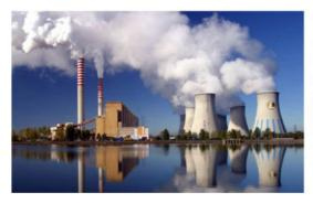
The **Belchatów Power Station** is a large 5298 MW lignite-fired power station situated near Belchatów in Łódź Voivodeship. It is the largest thermal power station in Europe, and fourth largest fossil fuel power stations in the world. Units: 12 x 370 MW 1 x 858 MW (supercritical)
