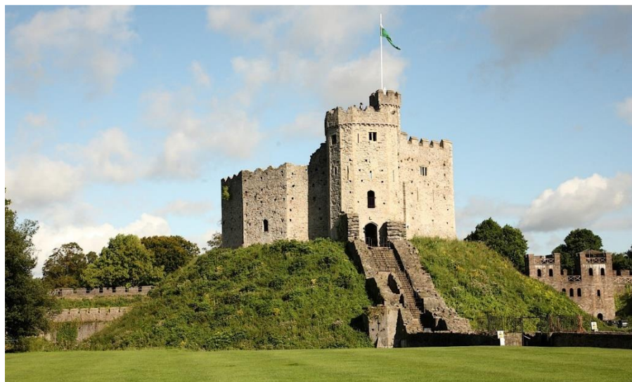
Picture 9 – Cardiff Castle (Source: cardiffphotos.co.uk)
