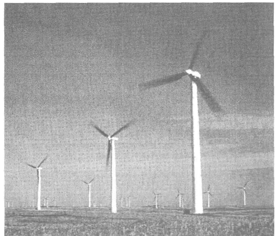
Fig. 1 Wind farm in the midwestern United States. (Courtesy of Enron Corp.)
