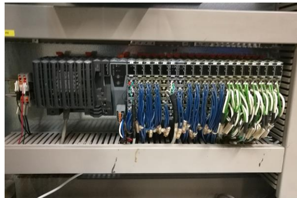
Fig.2: PLC – programmable logic controller, in this case control system of an reflow oven
