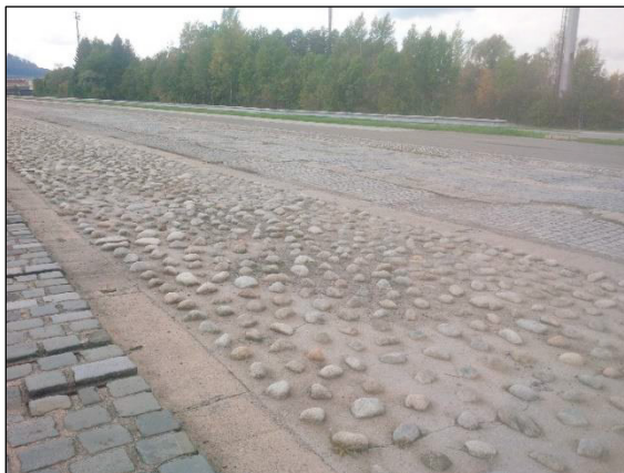
Fig. 5. Special roads at testing grounds.
