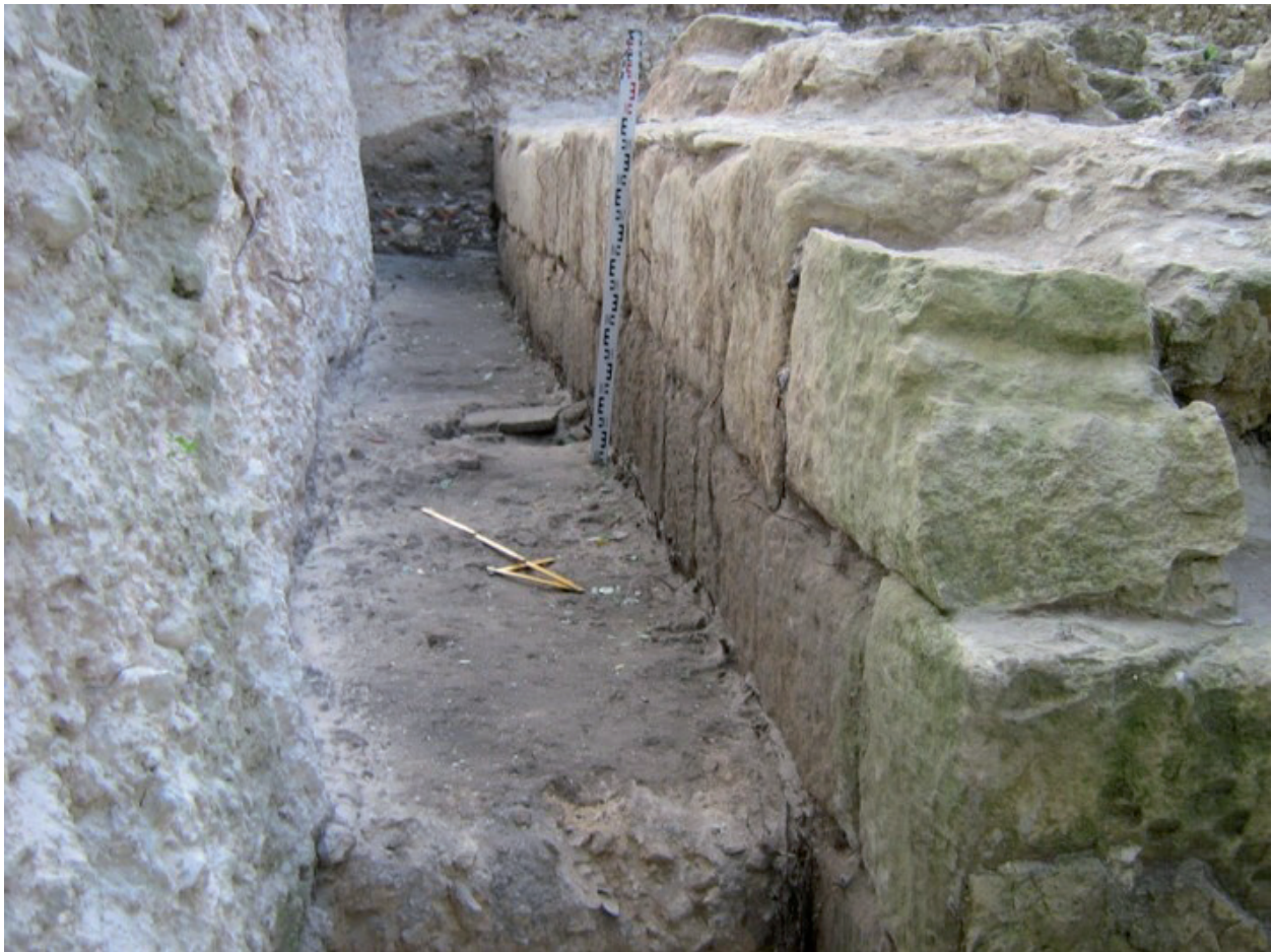
Fig. 7. Pińczów, SE tower wall face made of sandstone blocks. A. Andrzejewski.
