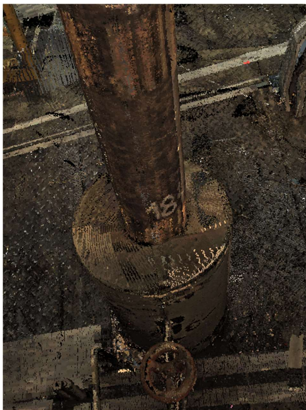
Obr. 2: Potrubí Bypassu \varnothing 157 \times 18
